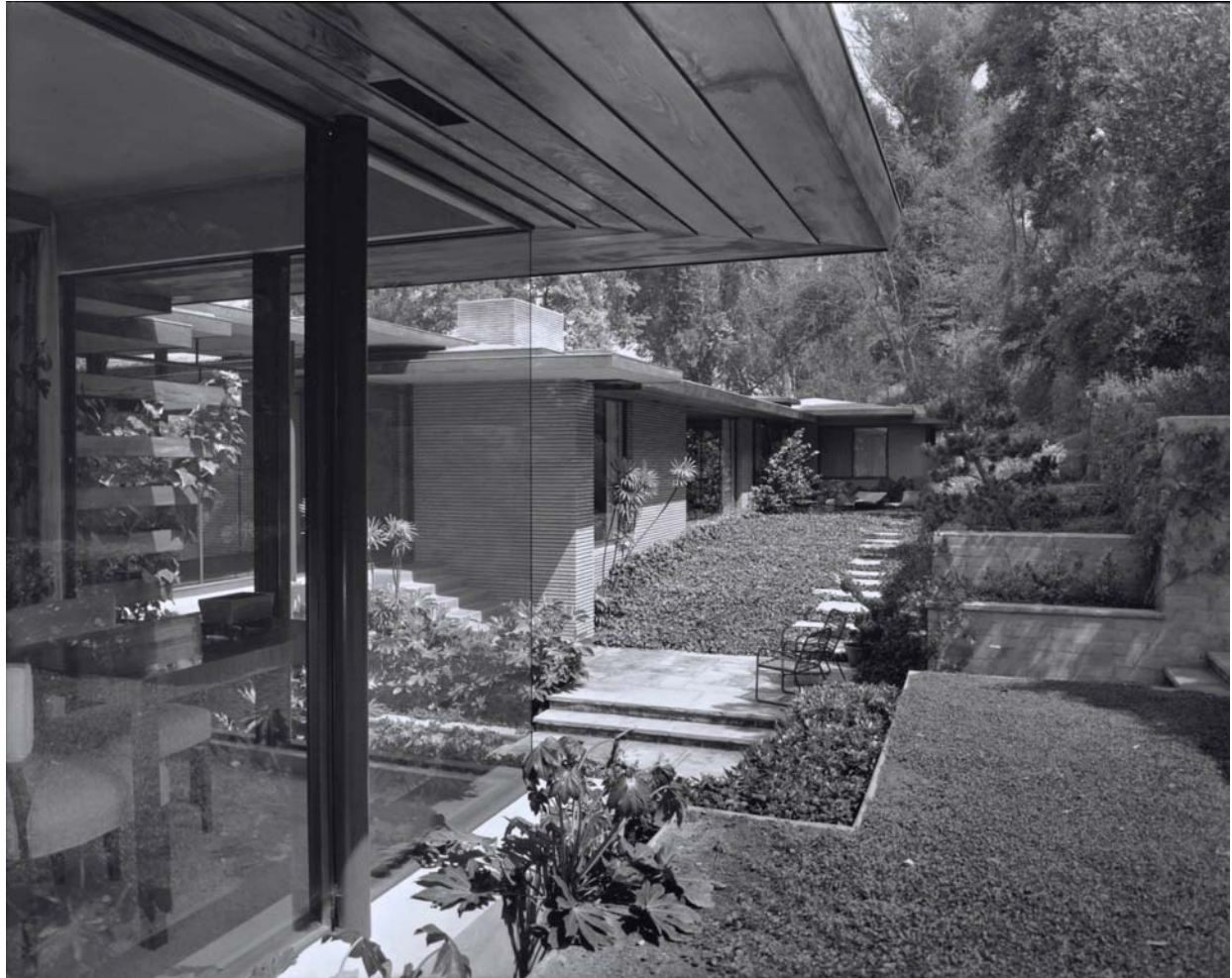
Figure 9. Lyon House, east and north façades, view facing northwest. Photograph by Julius Shulman, 1951. © J. Paul Getty Trust. Getty Research Institute, Los Angeles [2004.R.10(Job 958)].
